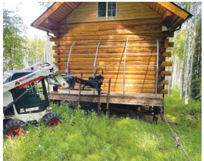
Helical Piers save a beautiful cabin!
