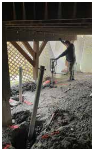
New support for deck by the river
